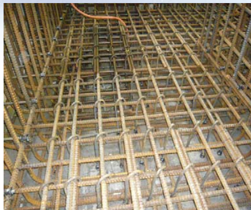
PLATE-NUT METHOD (SLAB)
